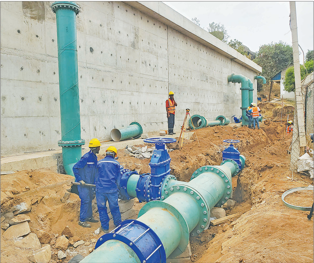
WATER technicians undertake construction work on a water substation at Sahwa, Lwahnima Ward, Nyamagana District in Mwanza, yesterday. The facility is expected to become operational in December. (Photo by Abela Msikula)
